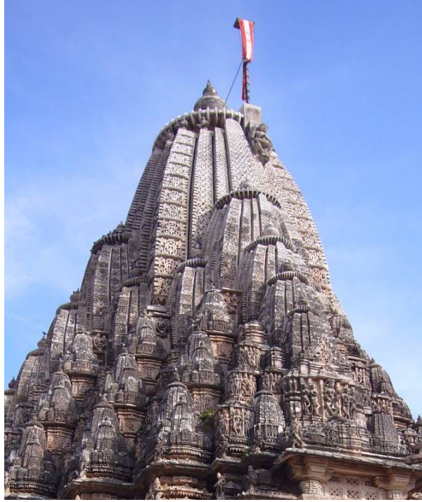
Figure 8. Taranga, view of the śikhara from the North West, with āmalasāra , kalaśa and dhvaja . Photo: Author, 2007.
